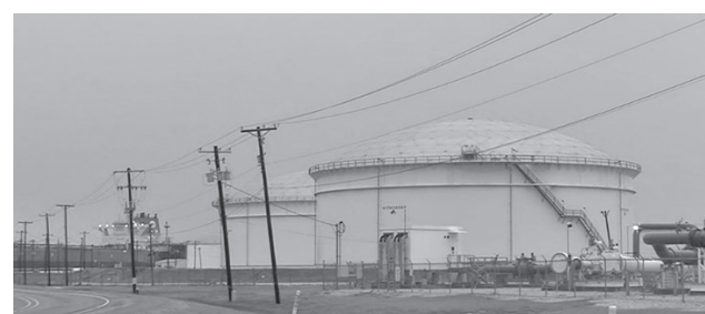
Courtesy: Desiree Beaudry An view of the energy export terminal formerly operated by MODA, purchased by Enbridge in 2021.
