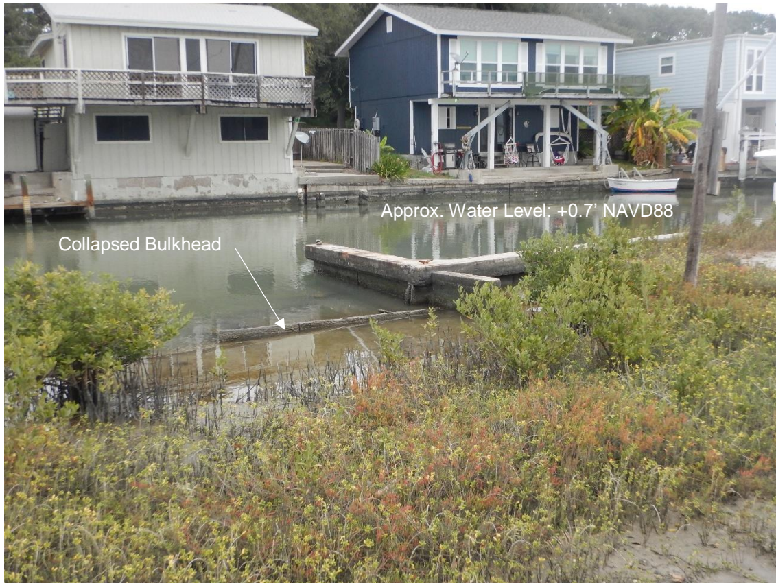
Figure 2. Failed Bulkhead
