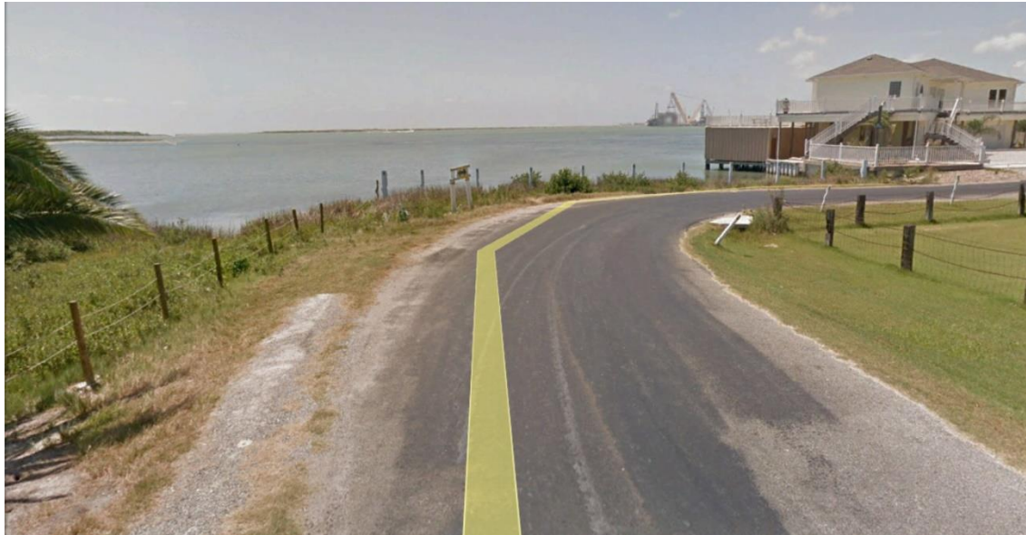
Figure 27. Unprotected shoreline adjacent to Post Oak Street and Inglewood Drive (Source: Google Earth)
