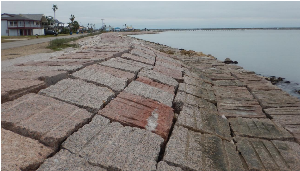
Figure 1. Ingleside Revetment along Bayshore Drive
